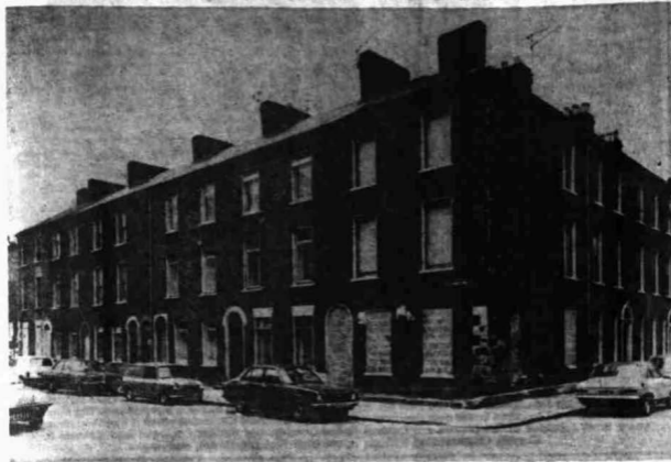
Some of the Georgian homes saved from demolition.
